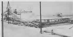
Lago's new sulfur handling facilities, with sulfur slaters in foreground and sulfur stacker to the left.
